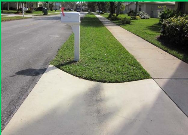
**A properly maintained swale. Note that only the driveway is paved.**
