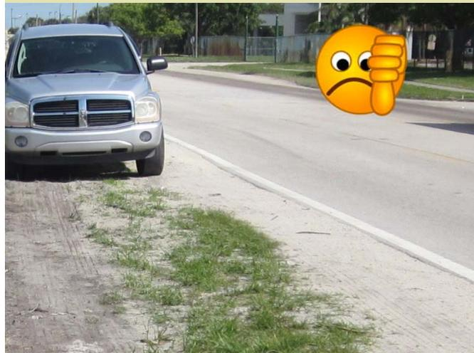
A poorly maintained swale. Note that the entire swale area is compacted due to vehicle parking.
