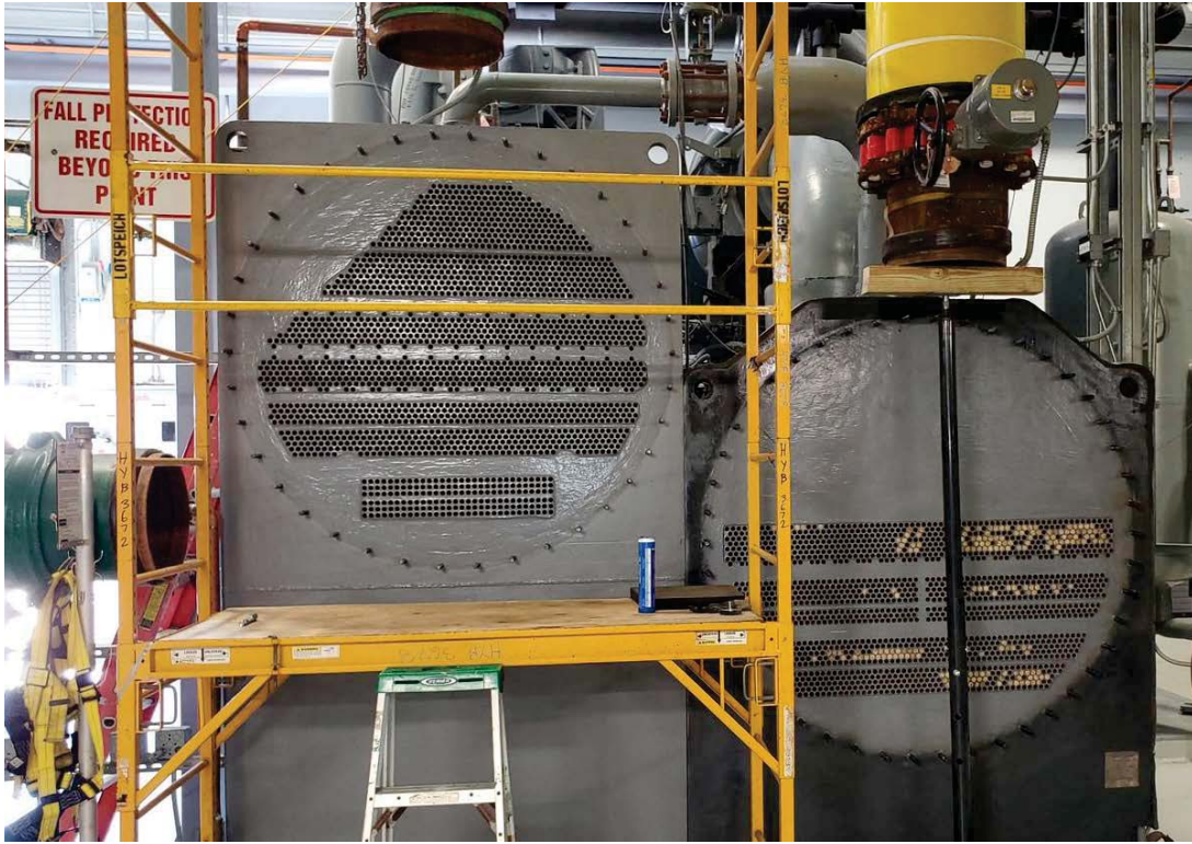
Chiller #2 Tube Sheets Following New Epoxy
