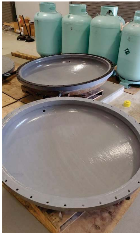
Chiller #2 End Bell Following New Epoxy
