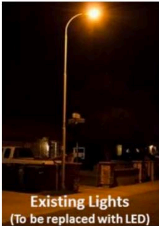
Existing 2200 Kelvin HPS
